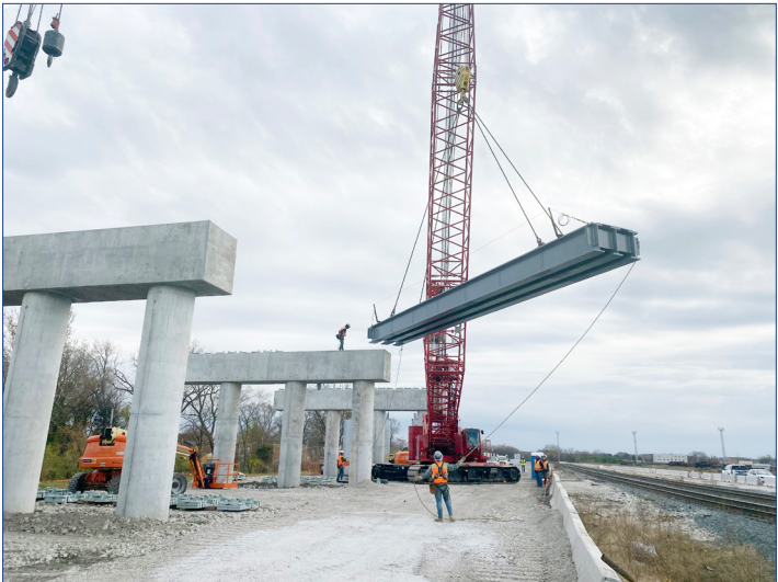
Construction team placing structural steel for the Forest Hill Flyover (P3) Project.
