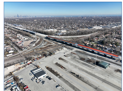
Forest Hill Flyover (P3) under construction.
